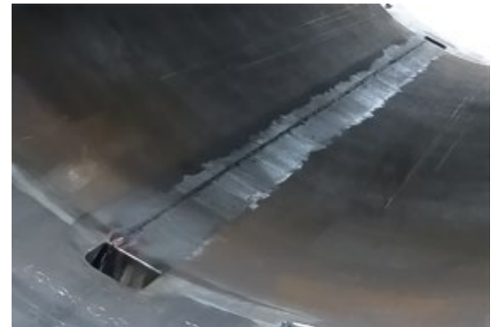
3m long 65mm thick welded in 11 minutes
