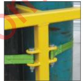
Cylinders secured by ratchet strap
